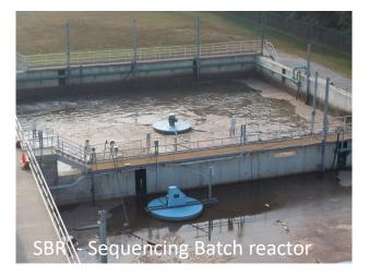
Upgrading the current lagoon system with a new space saving, cost effective, and efficient sequencing batch reactor system will improve energy efficiency, greatly reduce the possibility of equipment failures and allow the City to meet more stringent effluent limits anticipated in the future.
